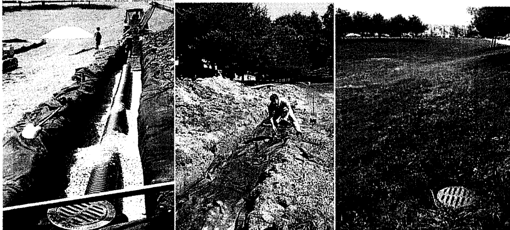
Figure 4: Example of Infiltration Trench Installation
